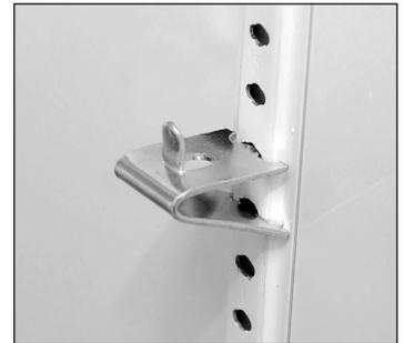
Fig. 9. Installed shelf clip.
