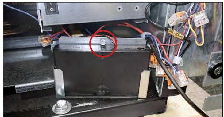
Fig. 3. Battery backup screw location.
